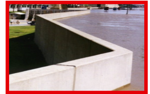
Figure 12 - Concrete sea wall (source: US Army Corps of Engineers)
