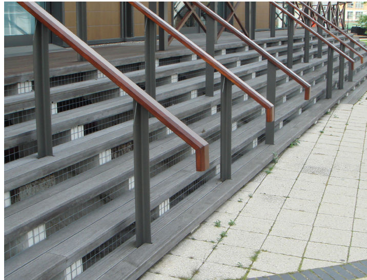
Figure 46 - Example of development locally raised above flood levels in Brentford, London (source: Baca Architects)
