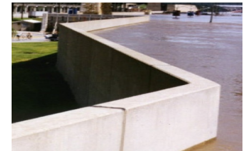
Figure 22 - Concrete sea wall (source: US Army Corps of Engineers)
