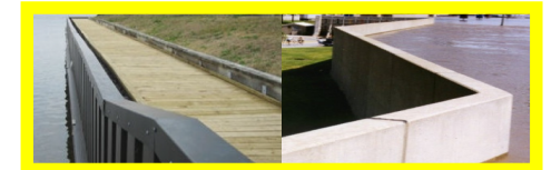
Figure 13 - Renovated piles with sea wall. (source: www.creativepultrusions.com ) Concrete sea wall (right)
