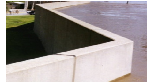
Figure 34 - Concrete sea wall (source: US Army Corps of Engineers)
