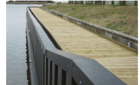
Figure 33 - Renovated piles (source: creativepultrusions.com)
