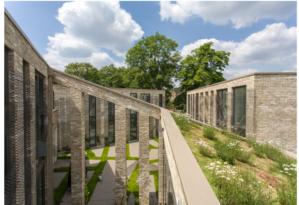
Figure 58 - Extensive wildflower and sedum green roof at Rockbourne Mews (source: R Barker, Baca Architects)
