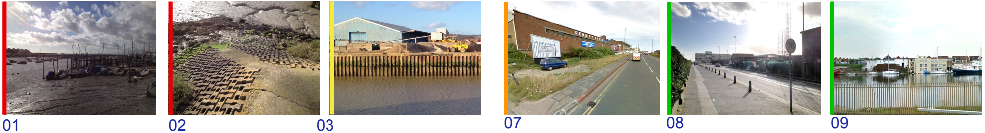
Figure 11 - Existing flood defences along the strategic sites 1 to 4 (plans using Google Earth Pro)
