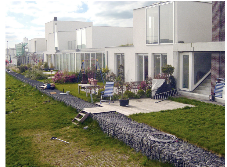
Figure 47 - Example of raised development in Ypenburg Netherlands (source: Baca Architects)
