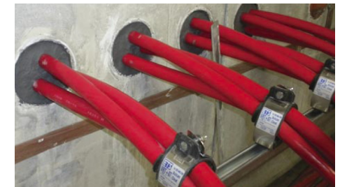
Figure 56 - Cable duct seal (source Aquobex)
