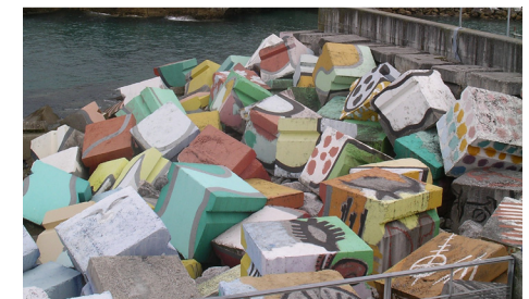
Figure 44 - Rock armour - Llanes Spain (source: Baca)
