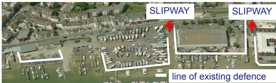
Figure 15 - Footbridge to Riverside centre, existing defences - (source: Bing Maps)
