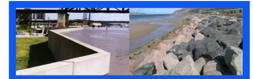
Figure 14 - Concrete sea wall (left) Natural rock armour (right) (© Jonathan Wilkins)
